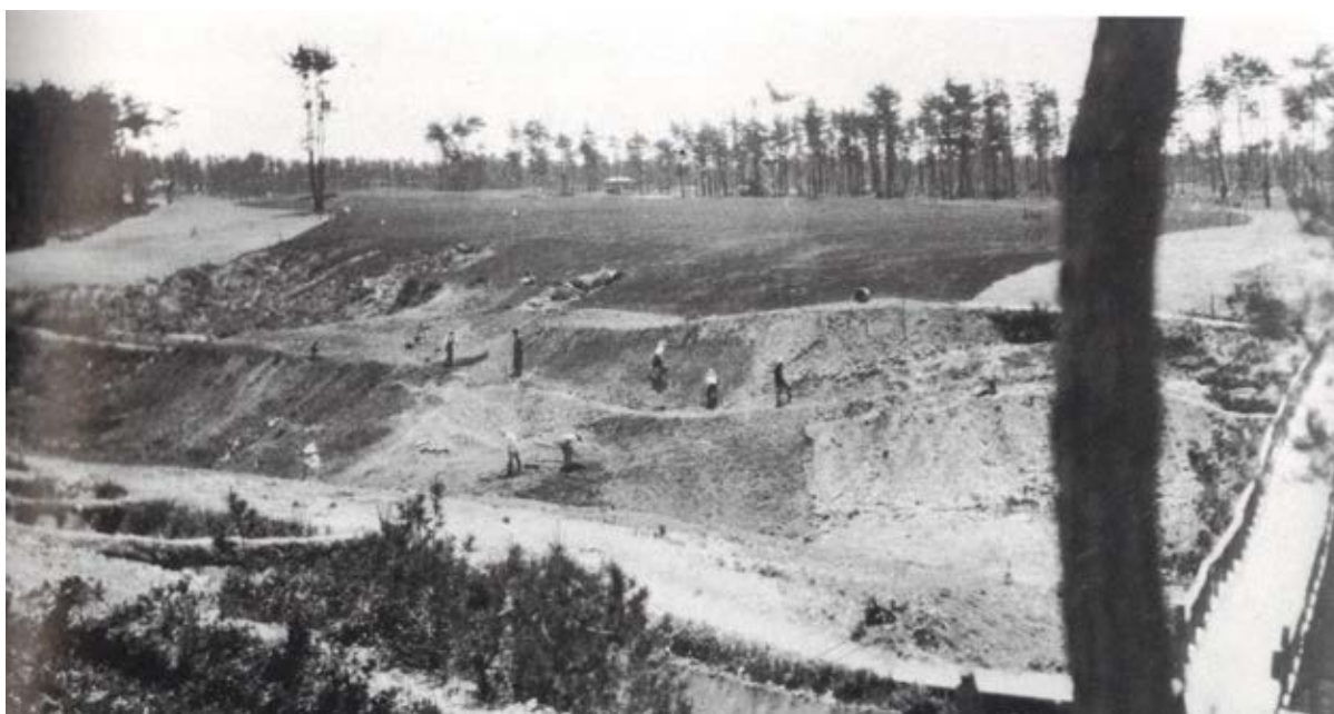
The 18 th hole under construction
