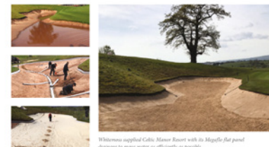
Whitemoss supplied Celtic Manor Resort with its MagaFlo flat panel drainage to move water as efficiently as possible
