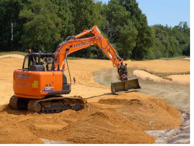
Fairways on the Kent layout have been capped with four inches of sand, as seen here on the fifteenth
