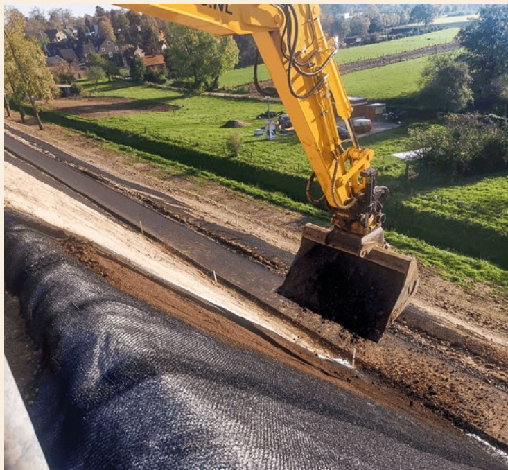
Turf reinforcement mat products provide lasting erosion control in the most challenging site conditions
